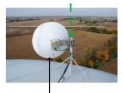
Opposite End: Saunders County Antenna Model: BHLP800-11-CR4 Antenna SN: 12US461720336 RFU Model: RFU-CX-11-Lz-TL RFU Serial: F453E10533 Centerline Height: 118' Azimuth: 290.12 deg. Frequency: 10875.000V/11365.000V
